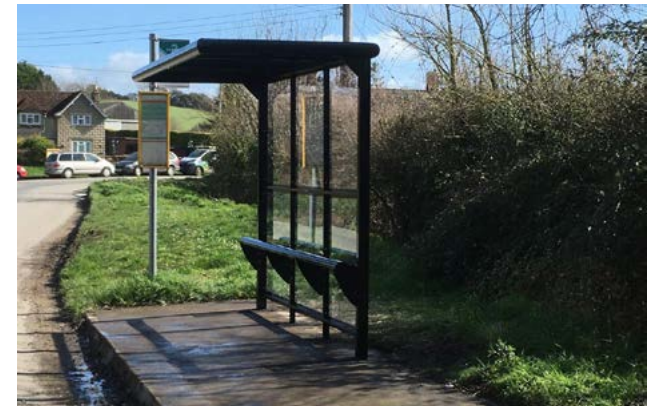
New bus shelter in Stockley
