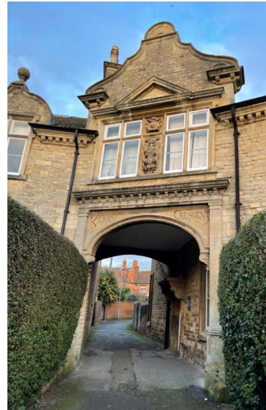
Kerry Crescent, Calne
