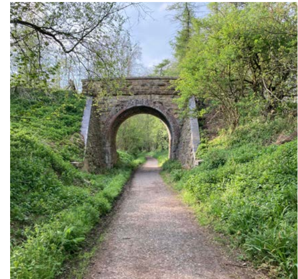
The Sustrans route along the River Marden Corridor
