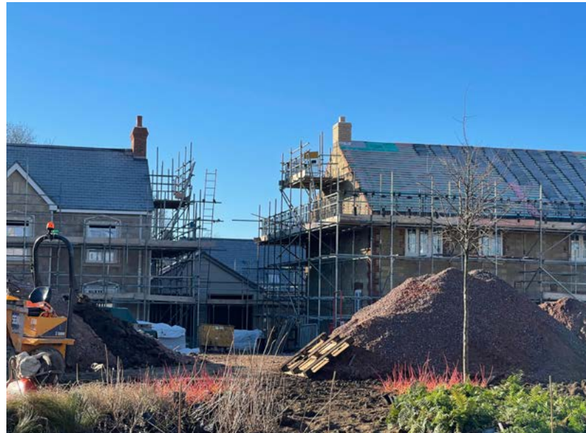
Houses under construction on Stoke Meadow
