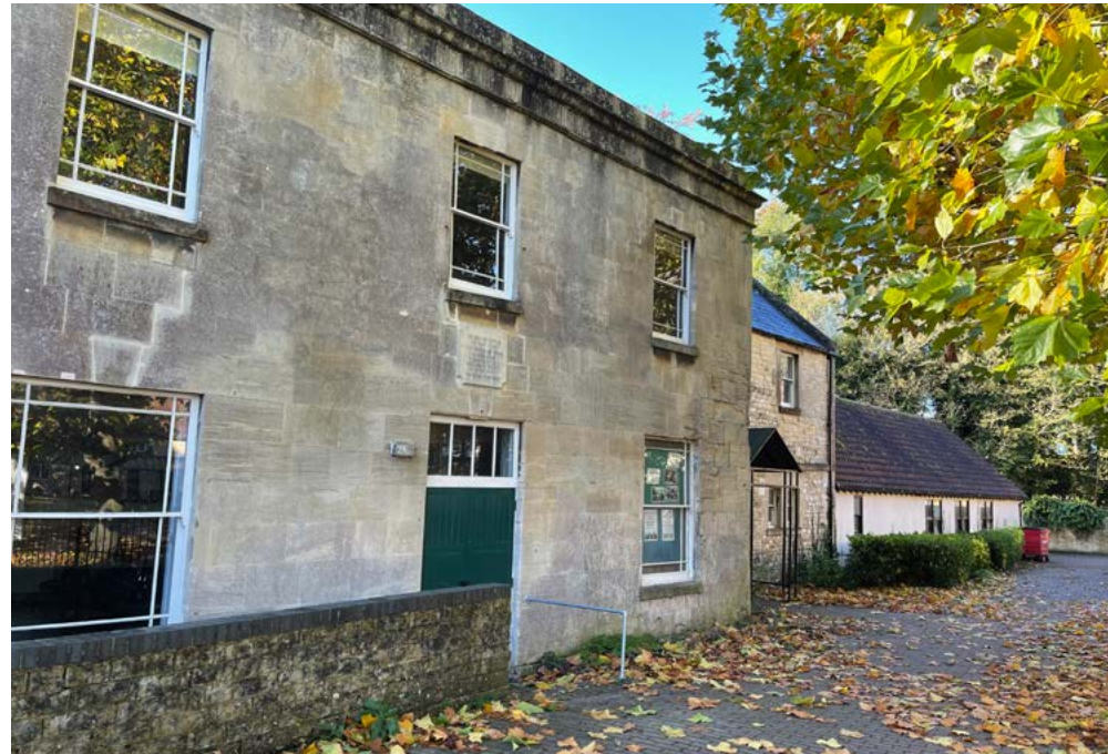
The Marden House Centre, Calne
