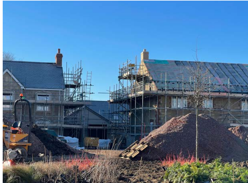
Houses under construction on Stoke Meadow
