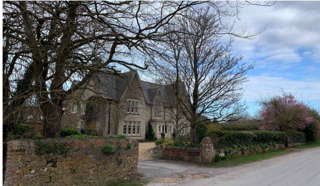
Calstone Manor Farm, Calstone
