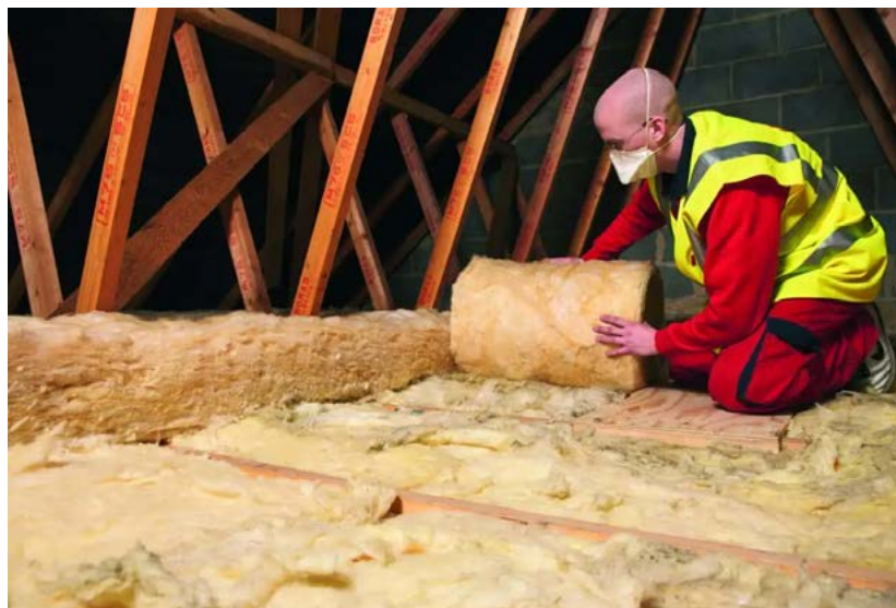
Installing loft insulation
