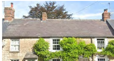
Gabled grey slate roofs on terraces, with local Bath Stone façade and climbing plants
