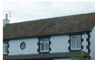
Gabled roof with red clay tiles
