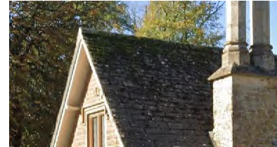
Gabled roof with grey slate tile
