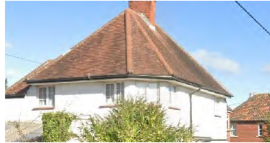
Hipped roof with red clay tiles and off-white render on the façade
