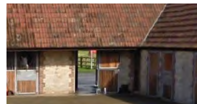
Gabled roof with red clay tiles and yellow stone and red brick
