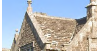
Cross-gabled roof with dark red slate
