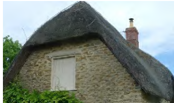
Mansard thatched roof
