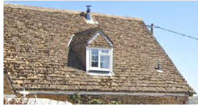
Gabled roof with red slate and gabled dormer with hung tiles
