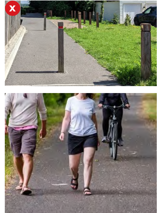
Figure 94: Examples of impermeable paving within rural settlements.
