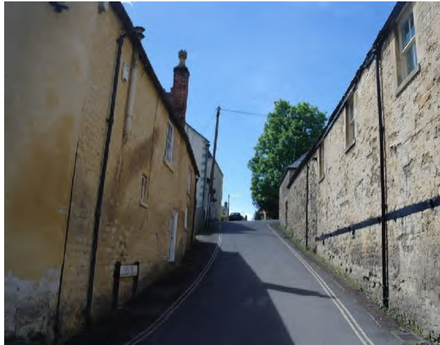
Figure 21: The hilly topography creates visual interest along the streetscape and pleasant evolving views and perspectives.
