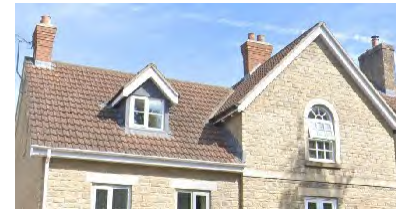
Gabled red clay pantile roof with exposed rubble façade and dormer window
