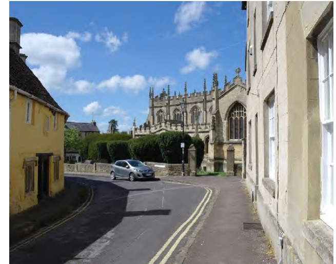
Figure 18: View towards the Grade I listed St Mary's Church, framed by C17 Almshouses along Kingsbury Street.
