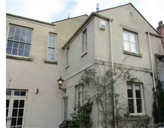
Figure 156: Positive local example of rear extension.
