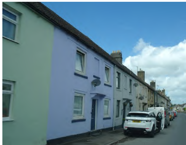
Figure 31: Photos taken along London Road showing both the consistent building lines and occasional building setbacks that allow for small-sized front gardens.
