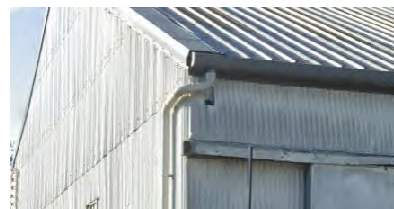
Gabled roof, off-white panelling
