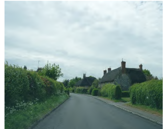
Figure 26: Properties are mostly set with a backdrop of the rural countryside in the Sandy Lane Conservation Area.
