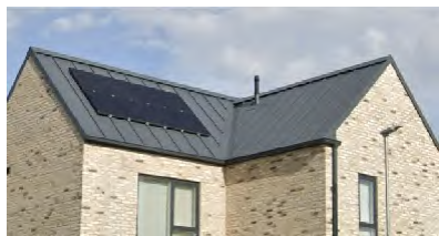
Grey slate roof with solar panels, buff brick façade
