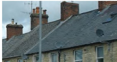
Gabled roof with grey slate tiles
