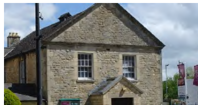
Exposed rubble stone
