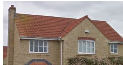
Gabled roof with red clay pantiles and local Bath stone on the façade
