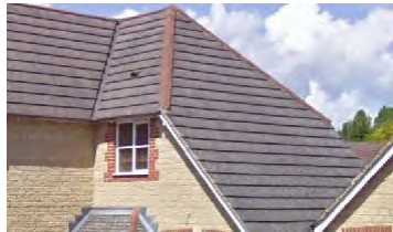
Cat-slide roof with grey tiles
