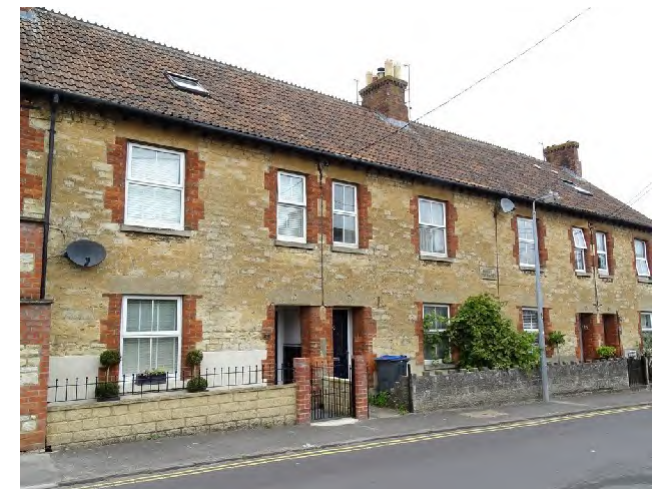
Figure 30: Terrace houses on Shelburne Road with Bath Stone facade and red brick decorative features.
