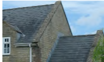
Gabled roof with grey slate
