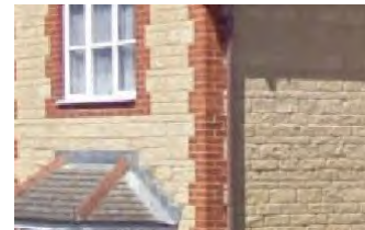
Rubble stone with red brick dressing
