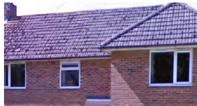
Cross-gabled roof with red clay tiles
