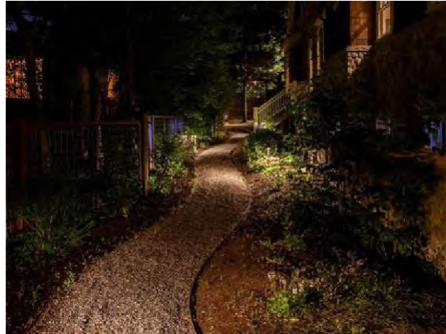
Figure 107: Example of path lighting where all lights are directed downwards, whilst the light sources are obscured.
