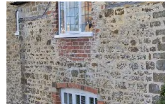
Exposed rubble with red brick dressing
