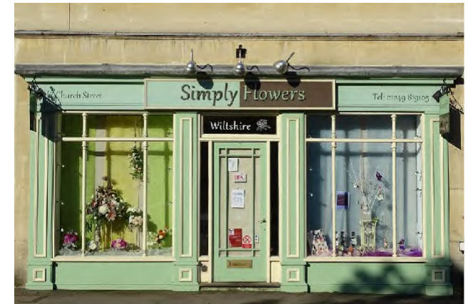
Figure 165: Positive local example of a shopfront with well-proportioned layouts and large windows facing onto the public realm, Church Street.
