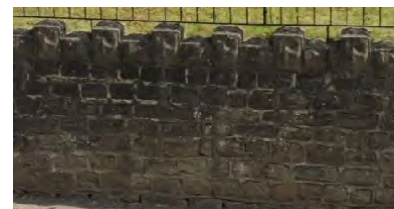
Low height stone wall with vertical coping stones
