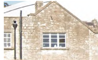
Gabled roof with clay tiles, stone façade
