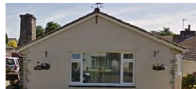
Painted façade with stone quoins and stone chimney on top of a gabled roof
