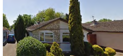
White-rendered façade with local stone and a variety of attractive planting on the front garden
