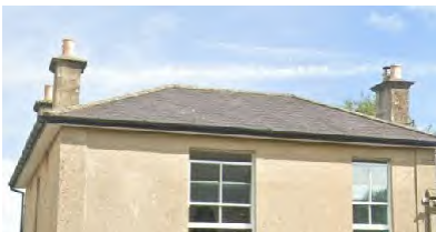
Grey slate hipped roof with stone façade
