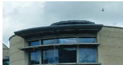
Flat roof with limestone ashlar on façade
