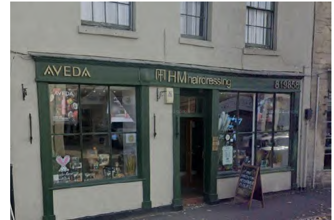
Figure 164: A local example of a well-laid out shopfront, with painted timber finished window and door frames, and clear signage positioned on fascia, Wood Street.
