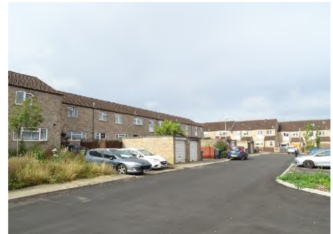
Figure 35: Houses laid out in clusters around the cul-de-sac of Woodroffe Square within the Coleman's Farm estate - another commonly recurring layout across this character area.
