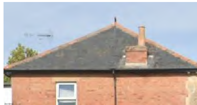
Hipped roof with grey slate and red clay ridges as well as red brick on the façade
