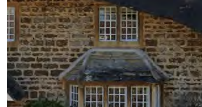
Local stone on façade
