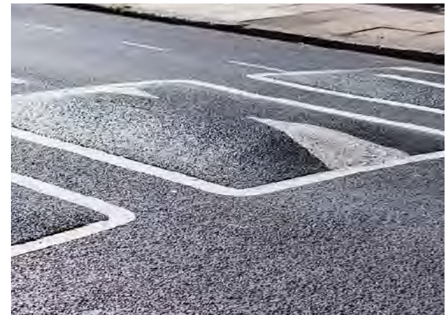
Figure 100: Example of a speed cushion.
