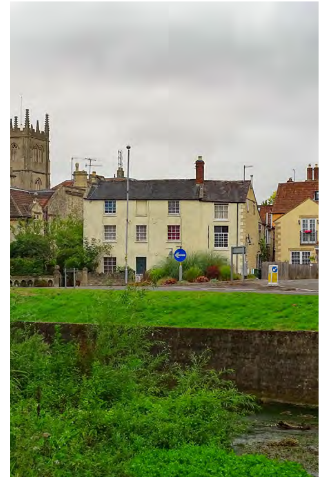
Figure 128: River Marden riverside walk - a part of green and blue corridor of the Calne area.
