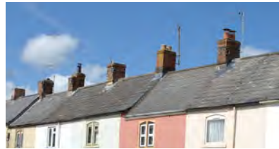
Roof with grey slates and red brick chimneys
