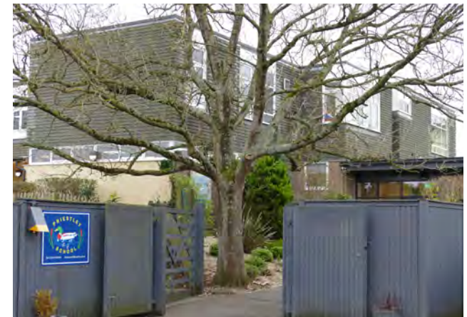
Figure 33: View of Priestley Primary School.
