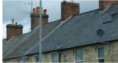
Gabled roof with grey slate tiles
