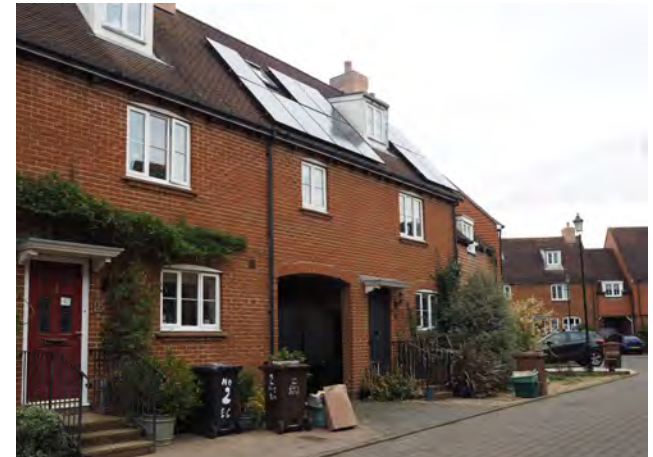
Figure 173: Local example in Ellis Close of implementing solar panels since the design stage.
