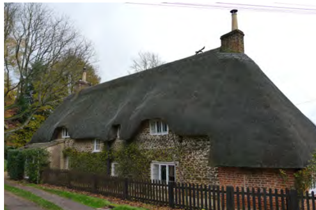
Figure 28: Houses with traditional ironstone façade and thatched roof found in Sandy Lane Conservation Area.
