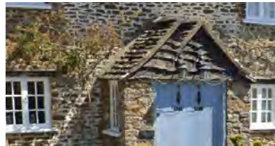
Gabled porch with dark coloured slate and black weatherboarding at the front
