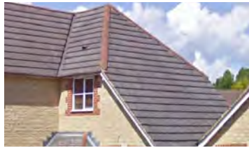
Cat-slide roof with grey tiles
