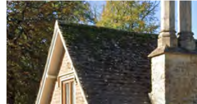
Gabled roof with grey slate tile
