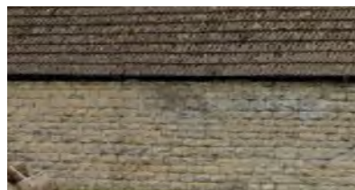
Local stone on façade
