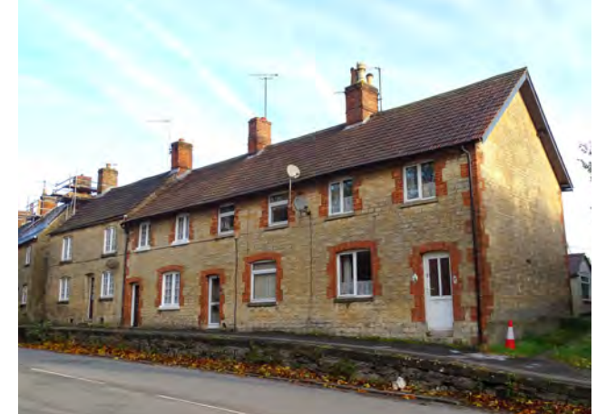
Figure 45: Row of terrace houses built with local stone and red brick dressing fronting onto Quemerford.
