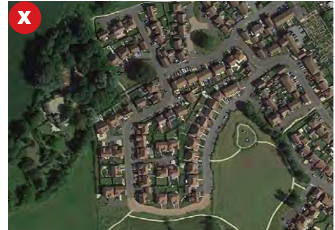
Figure 143: Local example of a recent development along Morgans Road with higher densities (~46-50 dph), creating abrupt edges that offer little opportunity for green spaces and buffers along the edges to allow for a smooth transition into the countryside.
