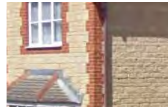
Rubble stone with red brick dressing
