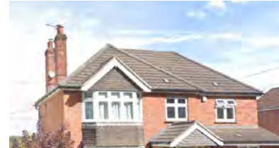
Clay tile hipped roof with red brick and hung tiles façade
