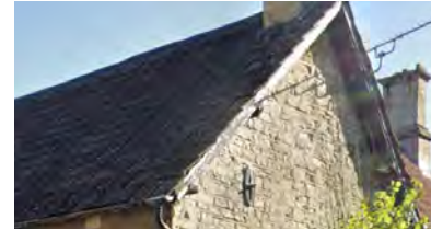
Gabled roof with grey slate and exposed rubble on the façade
