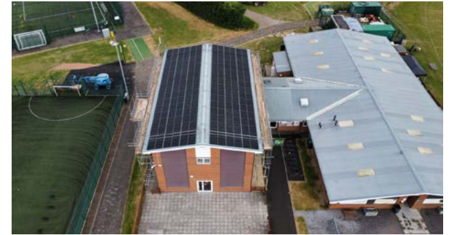
Beversbrook Sports Centre solar panels
