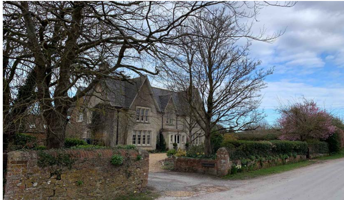
Calstone Manor Farm, Calstone
