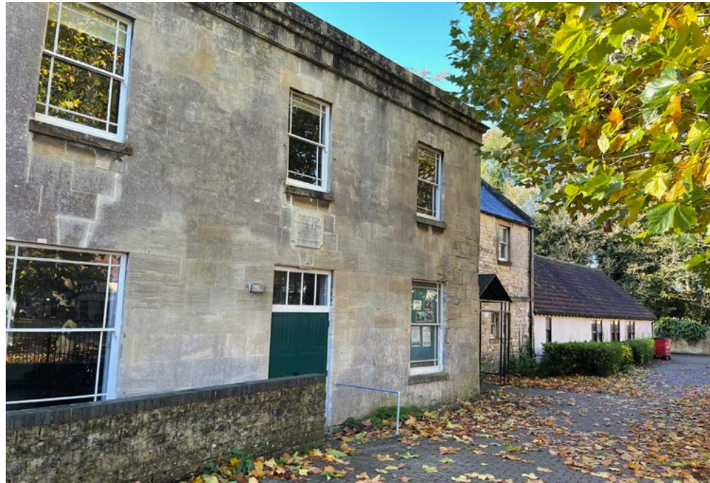
The Marden House Centre, Calne
