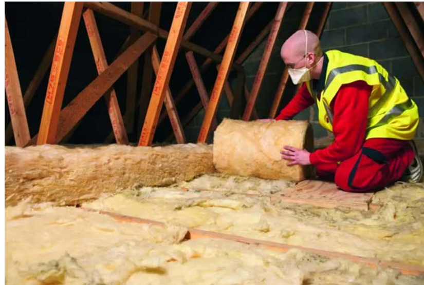
Installing loft insulation
