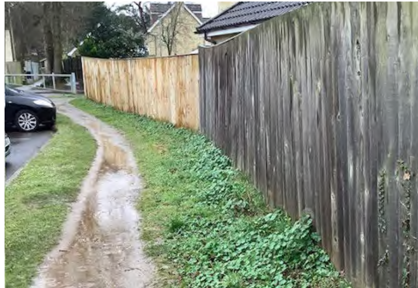
CALW65 links Derry Hill to NCN 403 - in need of an upgrade
