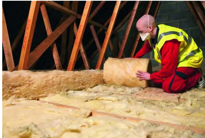
Installing loft insulation
