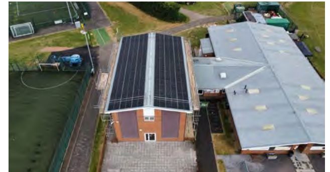
Beversbrook Sports Centre solar panels
