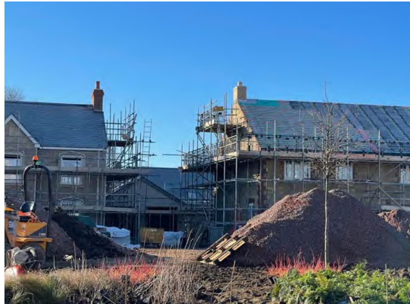
Houses under construction on Stoke Meadow
