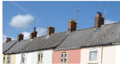
Roof with grey slates and red brick chimneys
