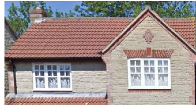
Red clay pantile gabled roof with chimney, local Bath stone façade with red brick dressing
