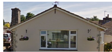
Painted façade with stone quoins and stone chimney on top of a gabled roof
