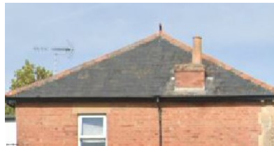
Hipped roof with grey slate and red clay ridges as well as red brick on the façade
