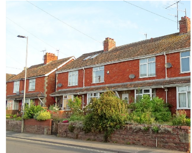
Figure 32: View along Oxford Road showing the linear layout of the buildings and the backdrop vegetation that add positively to the street scene.
