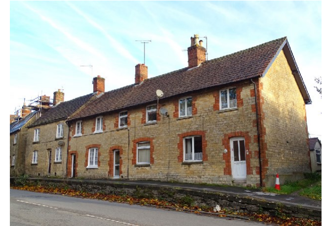
Figure 45: Row of terrace houses built with local stone and red brick dressing fronting onto Quemerford.
