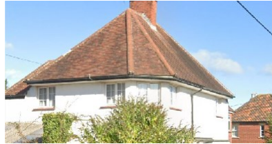
Hipped roof with red clay tiles and off-white render on the façade
