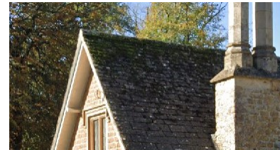
Gabled roof with grey slate tile
