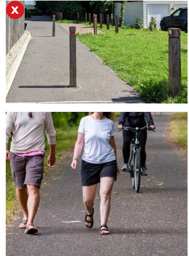
Figure 94: Examples of impermeable paving within rural settlements.
