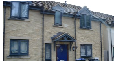
Stone façade with gabled tile roof and dormer windows
