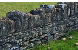
Low height stone wall with vertical coping stones
