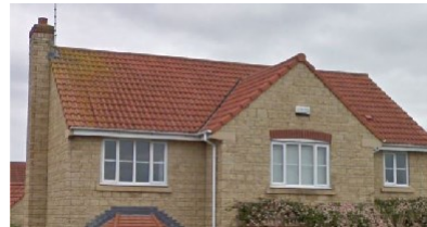
Gabled roof with red clay pantiles and local Bath stone on the façade
