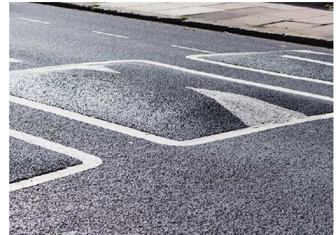
Figure 100: Example of a speed cushion.
