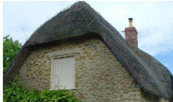
Mansard thatched roof
