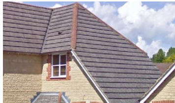
Cat-slide roof with grey tiles
