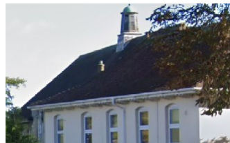
Clay tile gabled roof with decorative chimney and white-rendered façade
