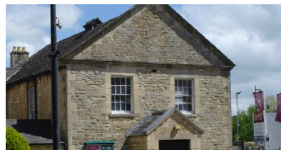
Exposed rubble stone
