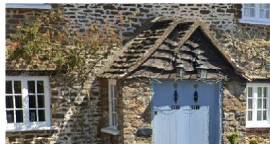
Gabled porch with dark coloured slate and black weatherboarding at the front
