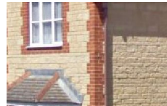
Rubble stone with red brick dressing
