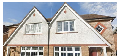
Double gabled roof with white render and buff brick façade
