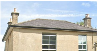
Grey slate hipped roof with stone façade
