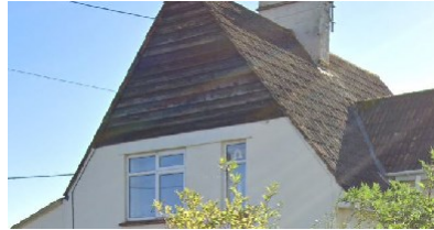
Dutch roof with grey slate and half black weatherboarding and half white render on façade
