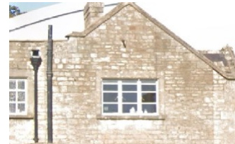
Gabled roof with clay tiles, stone façade
