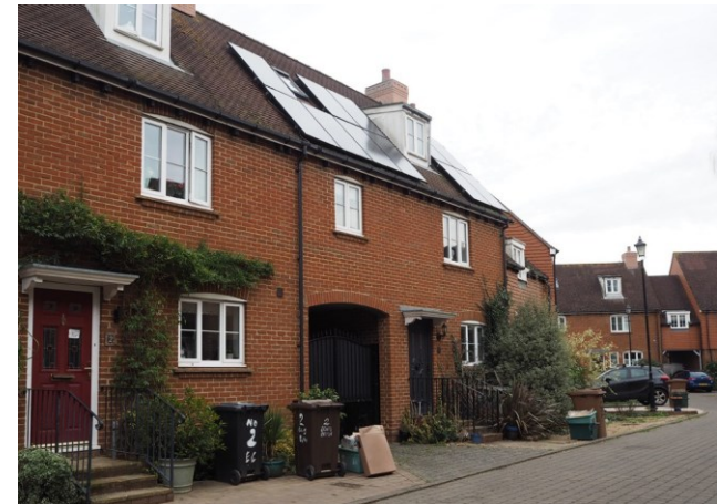
Figure 173: Local example in Ellis Close of implementing solar panels since the design stage.
