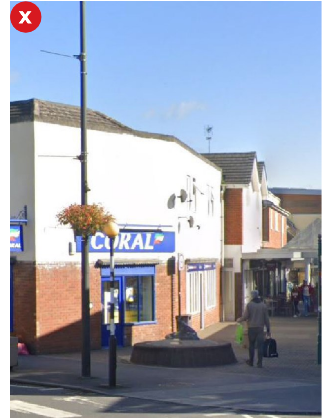
Figure 88: The red brick façades used at the corner buildings that lead to Phelps Parade create a less attractive street compared to the surrounding buildings. This is considered a poor design locally and should not be a model for future development in the area.
