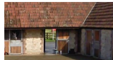
Gabled roof with red clay tiles and yellow stone and red brick
