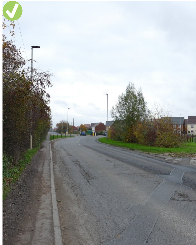
Figure 90: View along Oxford Road, where the industrial buildings are set back from the main road and screened with a landscape buffer. This buffer screens the industrial buildings offering pleasant views to the surrounding residential properties as well as reinforce the green feel of the area which is located in close proximity to the countryside. Hedgerow screening as shown demonstrates how industrial buildings are concealed from view in close proximity to residential areas.
