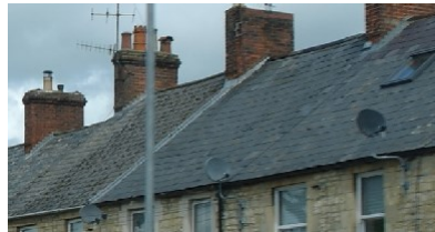
Gabled roof with grey slate tiles
