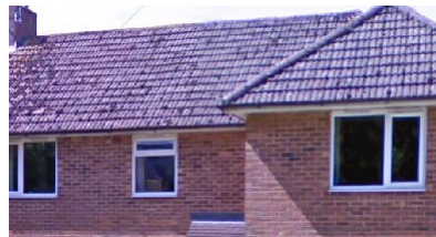
Cross-gabled roof with red clay tiles
