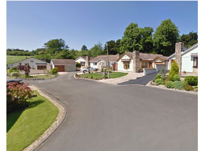
Figure 69: The 1-storey properties allow views to the background vegetation, whilst boundary treatments create clear delineations between public and private spaces, Walter Sutton Close.
