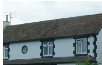
Gabled roof with red clay tiles
