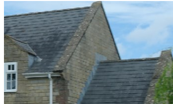
Gabled roof with grey slate
