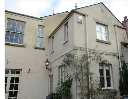
Figure 156: Positive local example of rear extension.
