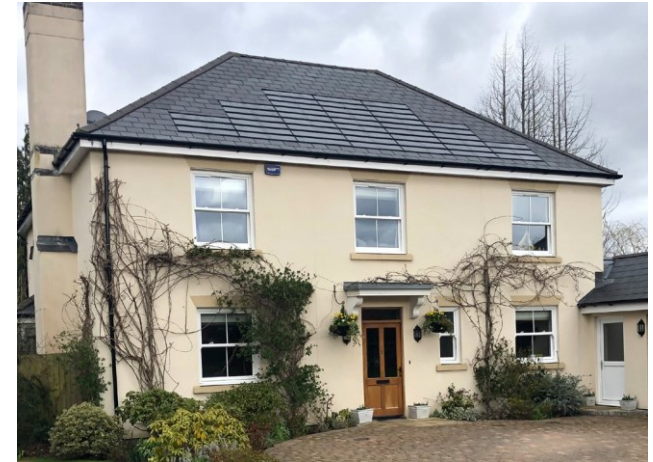
Figure 172: Use of shingle-like solar panels on a slate roof, with the design and colour of the solar panels matching those of the adjacent slate tiles.
