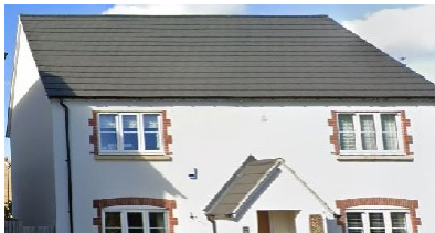
Grey slate roof with white-rendered façade and dormer porch
