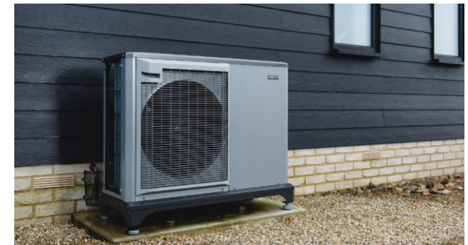
Figure 171: Example of an electric heat pump that is placed to the back of the house, whilst its grey colour fits nicely with the black weatherboarding of the property.
