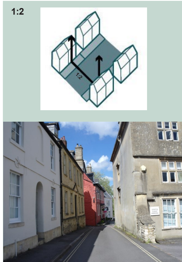
Figure 148: Local example of 1:2 enclosure, which is created by a narrow road in Calne town's medieval core bordered by houses on both sides of the road and narrow pavements.
