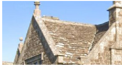
Cross-gabled roof with dark red slate
