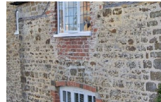
Exposed rubble with red brick dressing
