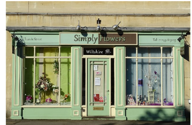
Figure 165: Positive local example of a shopfront with well-proportioned layouts and large windows facing onto the public realm, Church Street.
